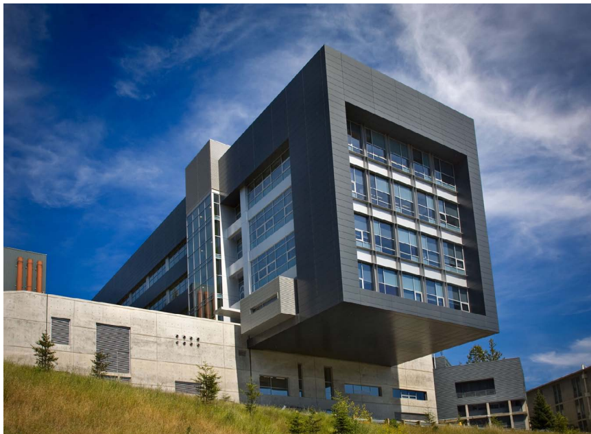
Molecular Foundry Building. Lawrence Berkeley Laboratory
