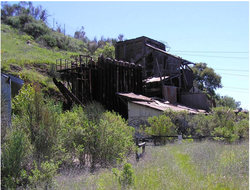
Ruins of the rotary furnace and condensing system (retorts) in the New Almaden Quicksilver Park. A 100 ton furnace was originally installed 1940; however, it was too large and subsequently replaced by 50 ton furnace that was used until 1976. Photo by W.E. Motzer (April 2012).
